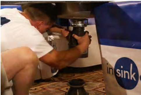
Jerry Peek gives one final twist during the Garbage Disposer Installation
